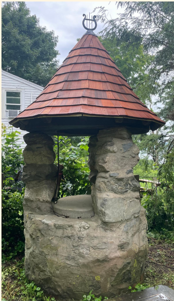
The new choir well roof was replaced by DND Construction out of Warren, Maine
